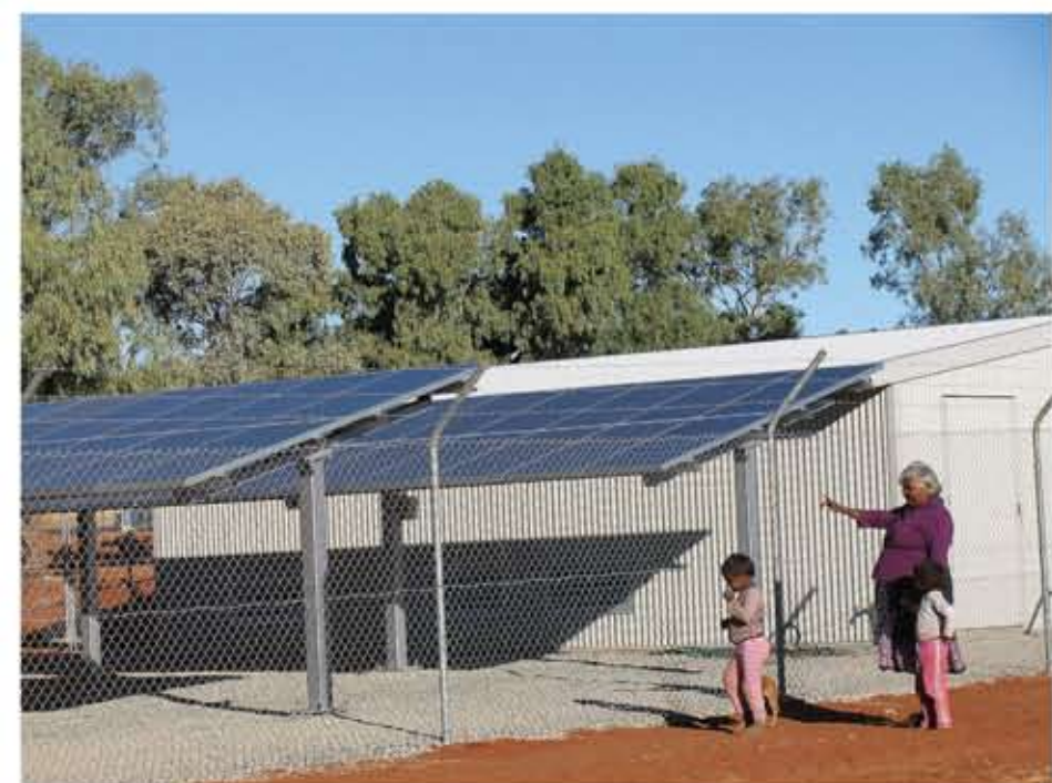
Solar arrays installed at Ulpanyali are part of a hybrid solar power system that is saving the community thousands of dollars.
