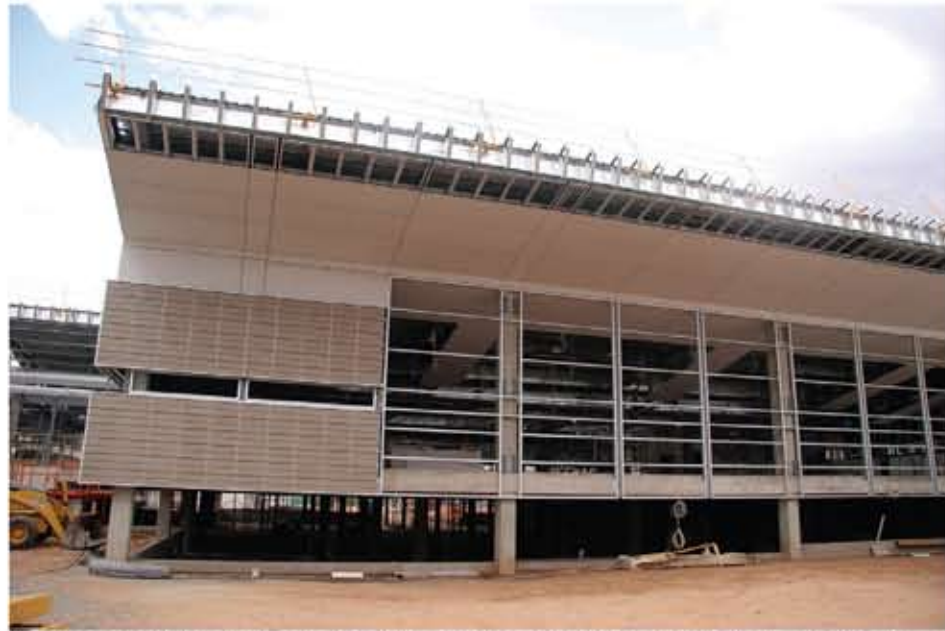
The north side of the new office while it was still under construction late last year.
