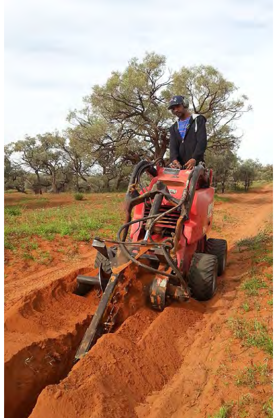
David Marshall digs a water line at Phillipson Bore outstation.
