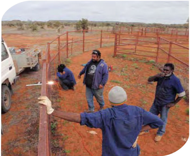
ABOVE: Tjuwanpa Rangers building stockyards, August 2010
