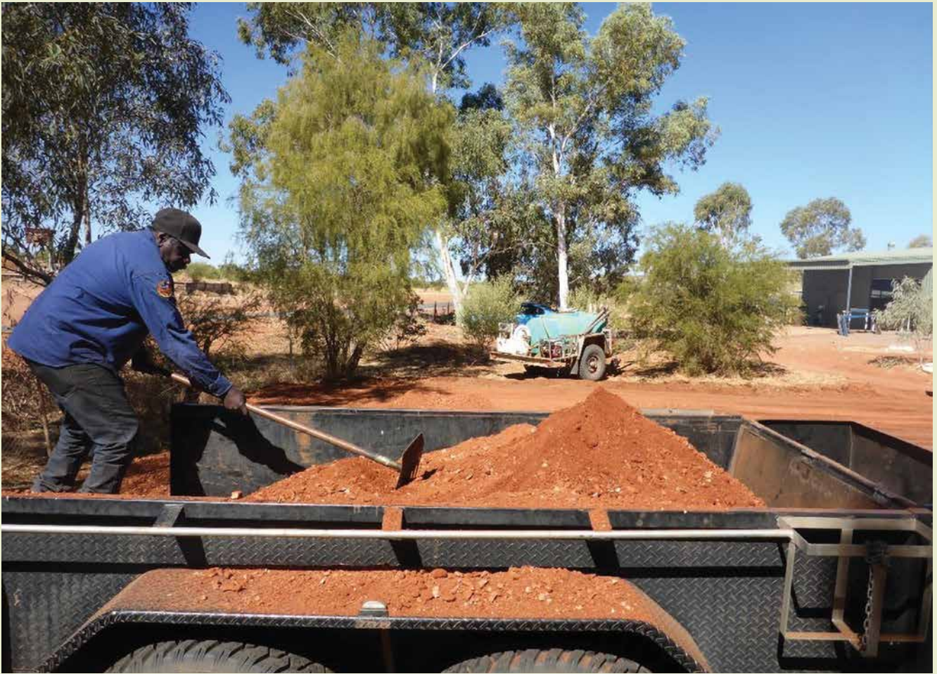
Christopher Ungwanaka working on new car park.
