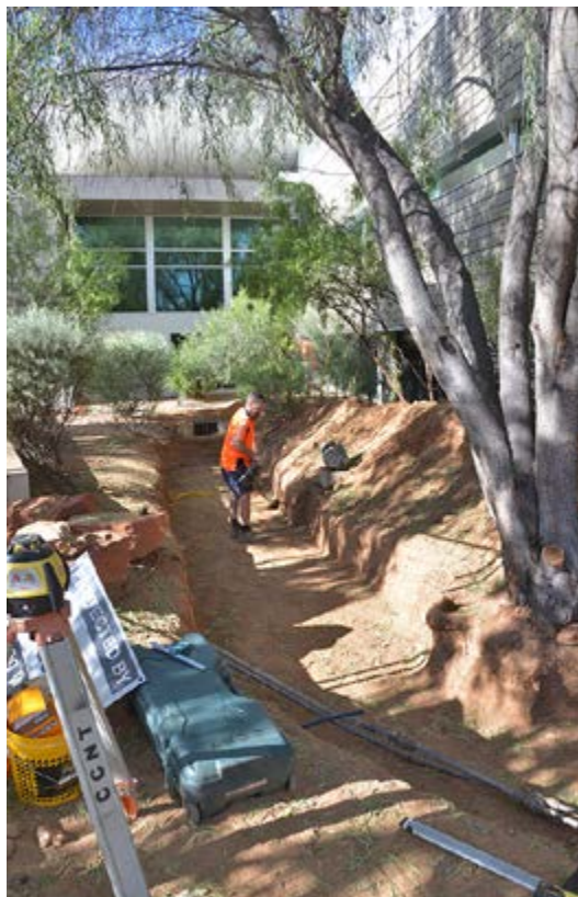
Before: Labourers dug trenches to divert rainwater from the CLC building in Alice Springs.
