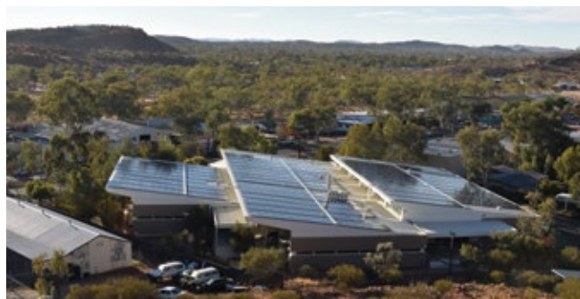
The new rooftop solar array includes a cloud camera that controls energy demand from the Alice Springs town grid.
