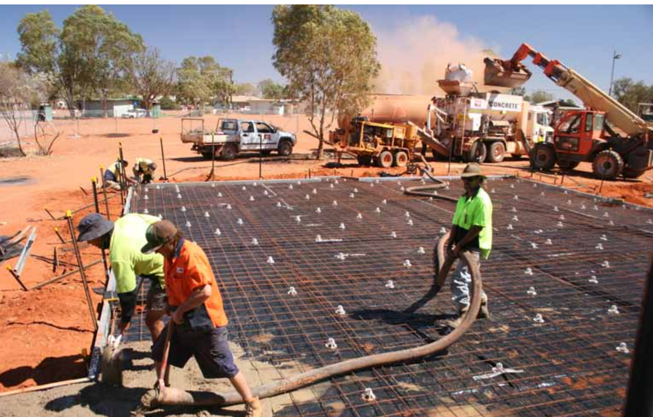
Pouring the slab for the Epenarra church extension – one of the community lease money projects completed in 2013.
