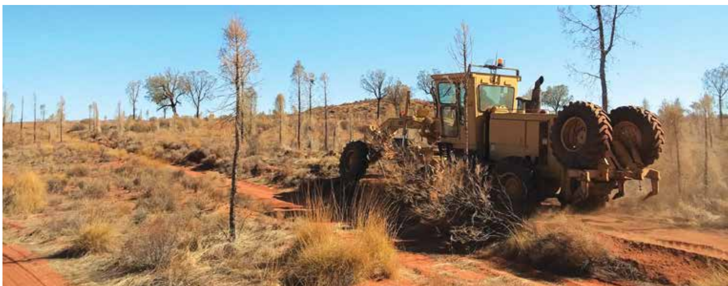
Backfilling erosion on the Kulpitjata track on the Kaṯiṯi Petermann IPA.
